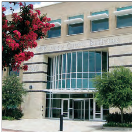
Eliminate Overspray on Buildings
